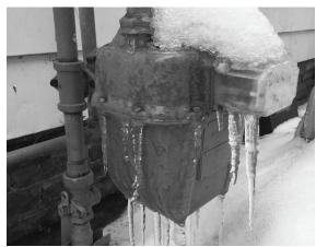
Natural gas meter equipment has a vent to regulate pressure. Snow that accumulates on or around the vent can obstruct the opening, creating a hazardous situation. Keep your family safe this winter by following these important steps:
